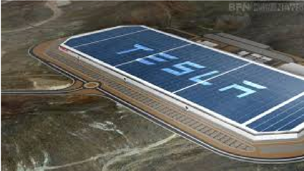
Figure 8.25: Tesla's Gigafactory 1 in Nevada produces improved lithium ion batteries. Energy for the factory is supplied by solar panels on the roof.
