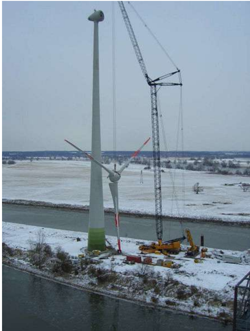
Figure 3.9: Erection of an Enercon E70-4 in Germany
