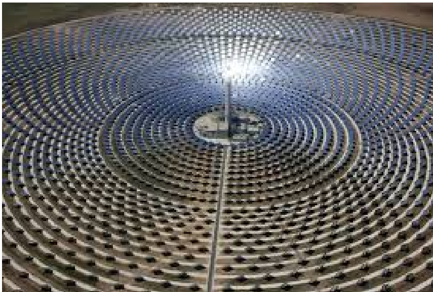
Figure 6.11: A solar thermal power plant. Arrays of heliostatic reflectors concentrate the sun's rays onto molten salt in the tower. The plant produces electricity at night because the salt remains hot..
