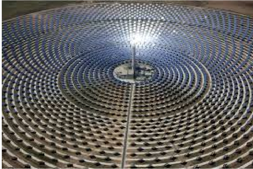
Figure 6.2: A solar thermal power plant. Arrays of heliostatic reflectors concentrate the sun's rays onto molten salt in the tower. The plant produces electricity at night because the salt remains hot..
