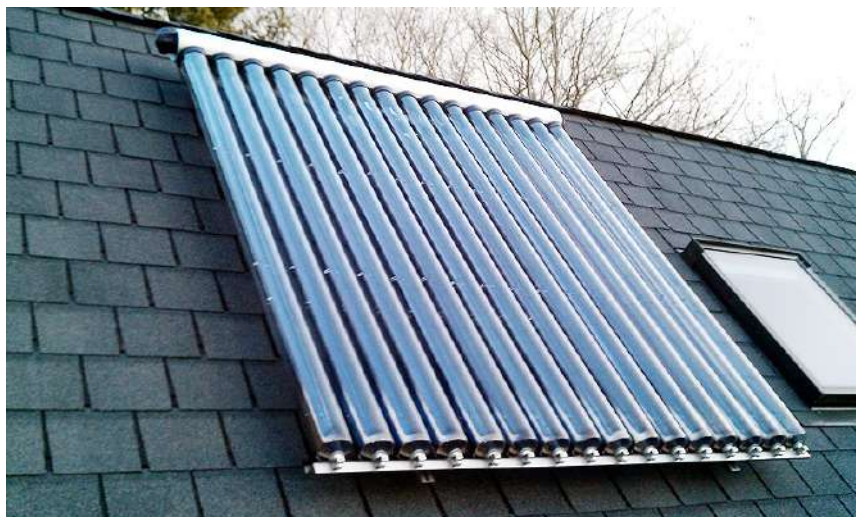
Figure 6.4: A rooftop solar thermal array for domestic water heating.
