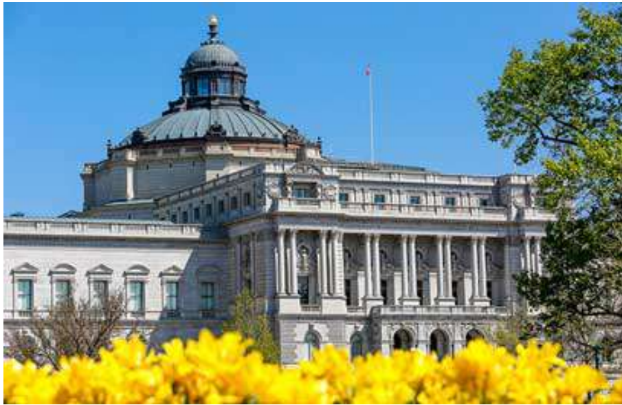
Figure 8.1: One of the three building which house the Library of Congress. It is the largest library in the world. More than 470 languages are represented in the library's book collection.
